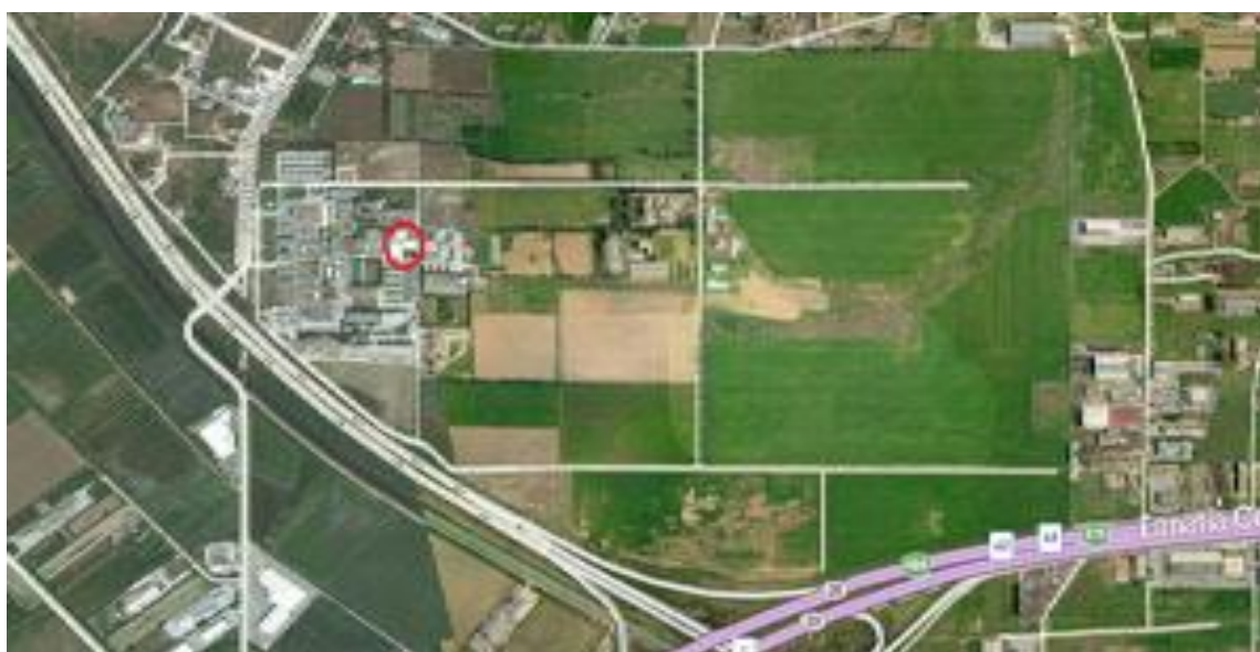
Figure 1. View of the Department's building
